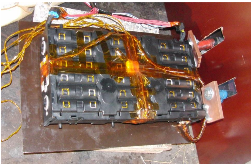
Figure 37. Module with electrical connection and thermal sensors before the test (Hybrid Commercial Vehicle (HCV)).
